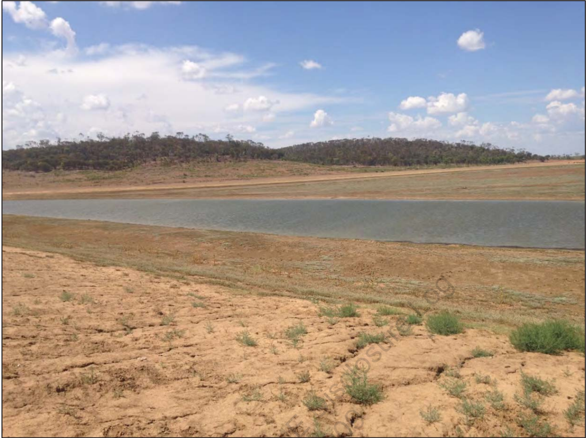
Plate 1-1: Two hillocks adjacent to the Belyando Junction Dam, providing a natural perimeter wall to the north of the storage.
