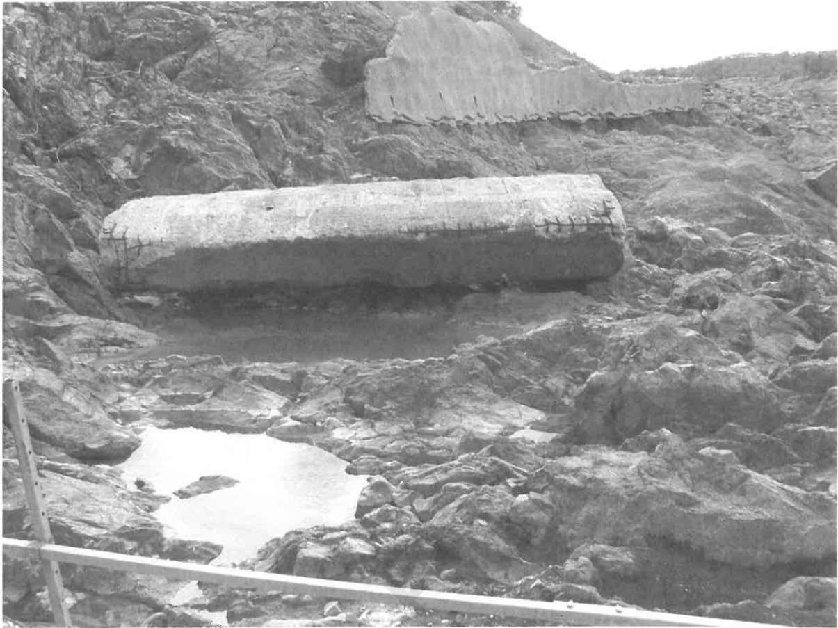
Photo 3 – Sill Block at Base of Left Abutment
