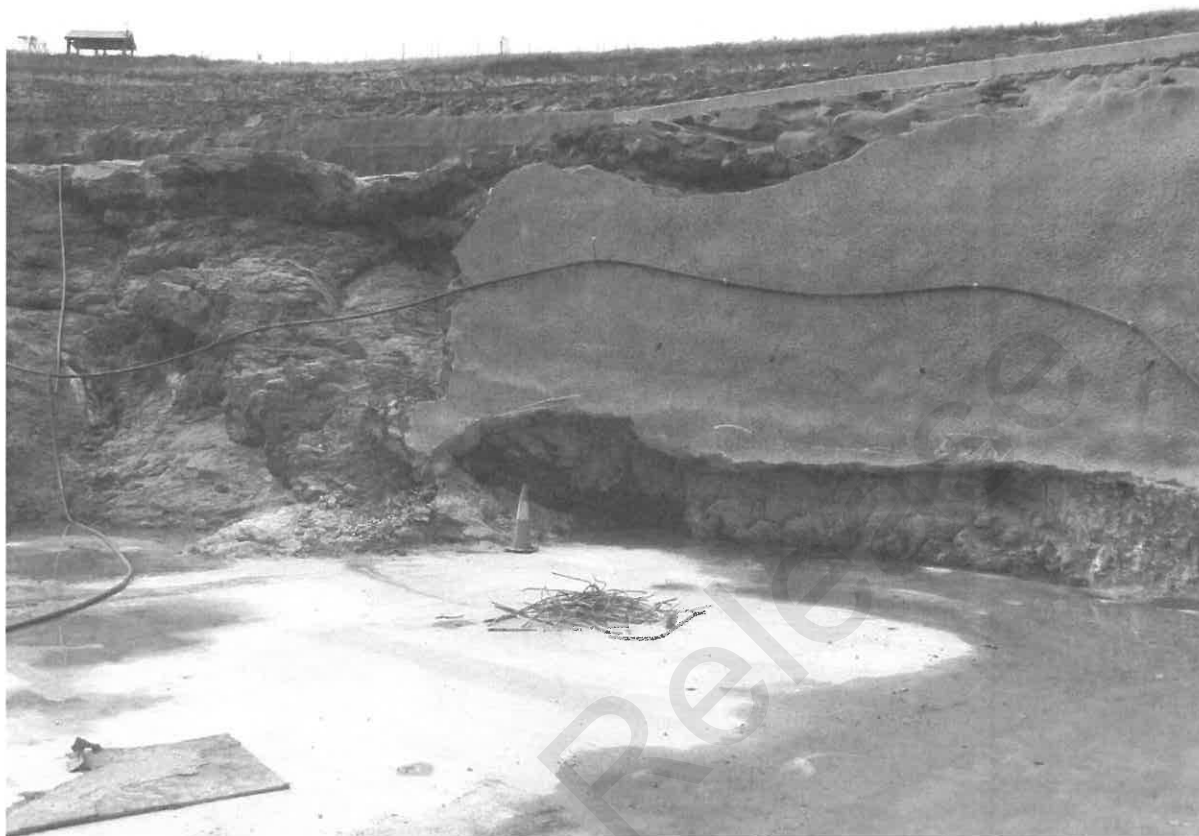
Photo 5 – Scour Hole at Right End of Apron Repaired
