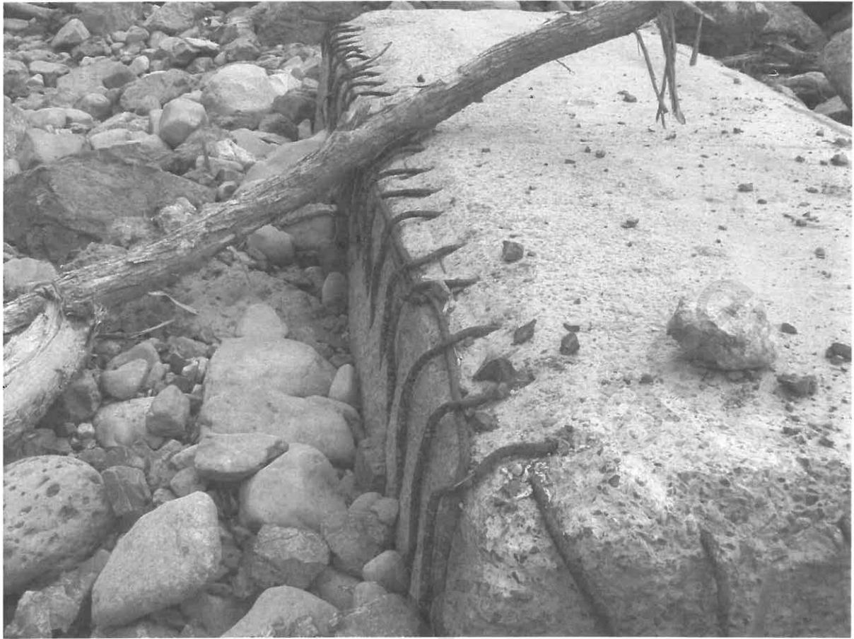
Photo 7 – A 7 tonne sill block carried 150m
