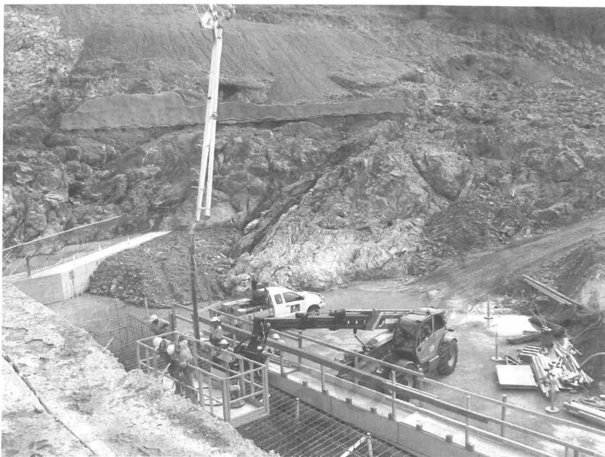
Photo 2 - Shear Feature (just right of concrete boom)
