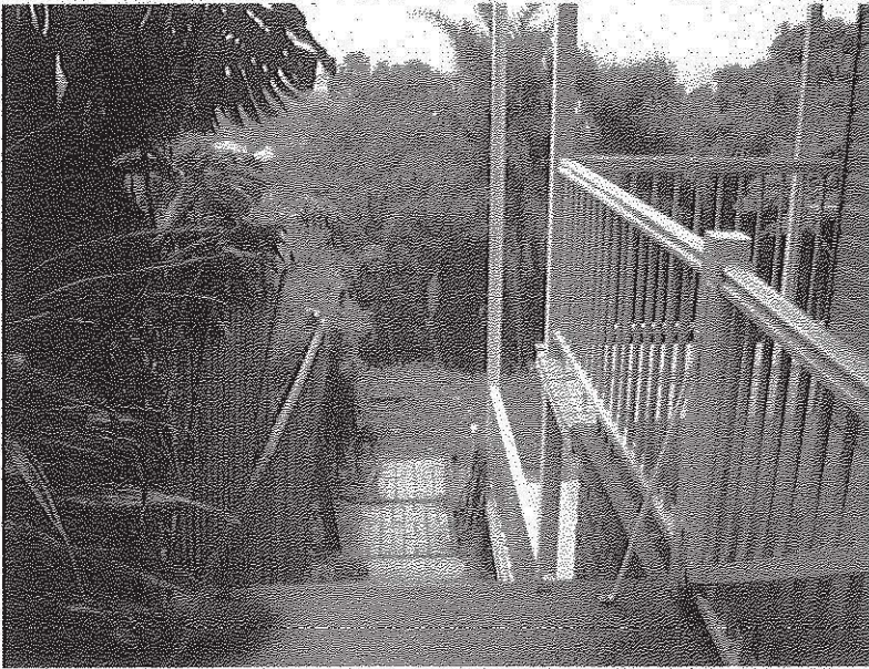
Photo of part of road closure looking down from laneway.
