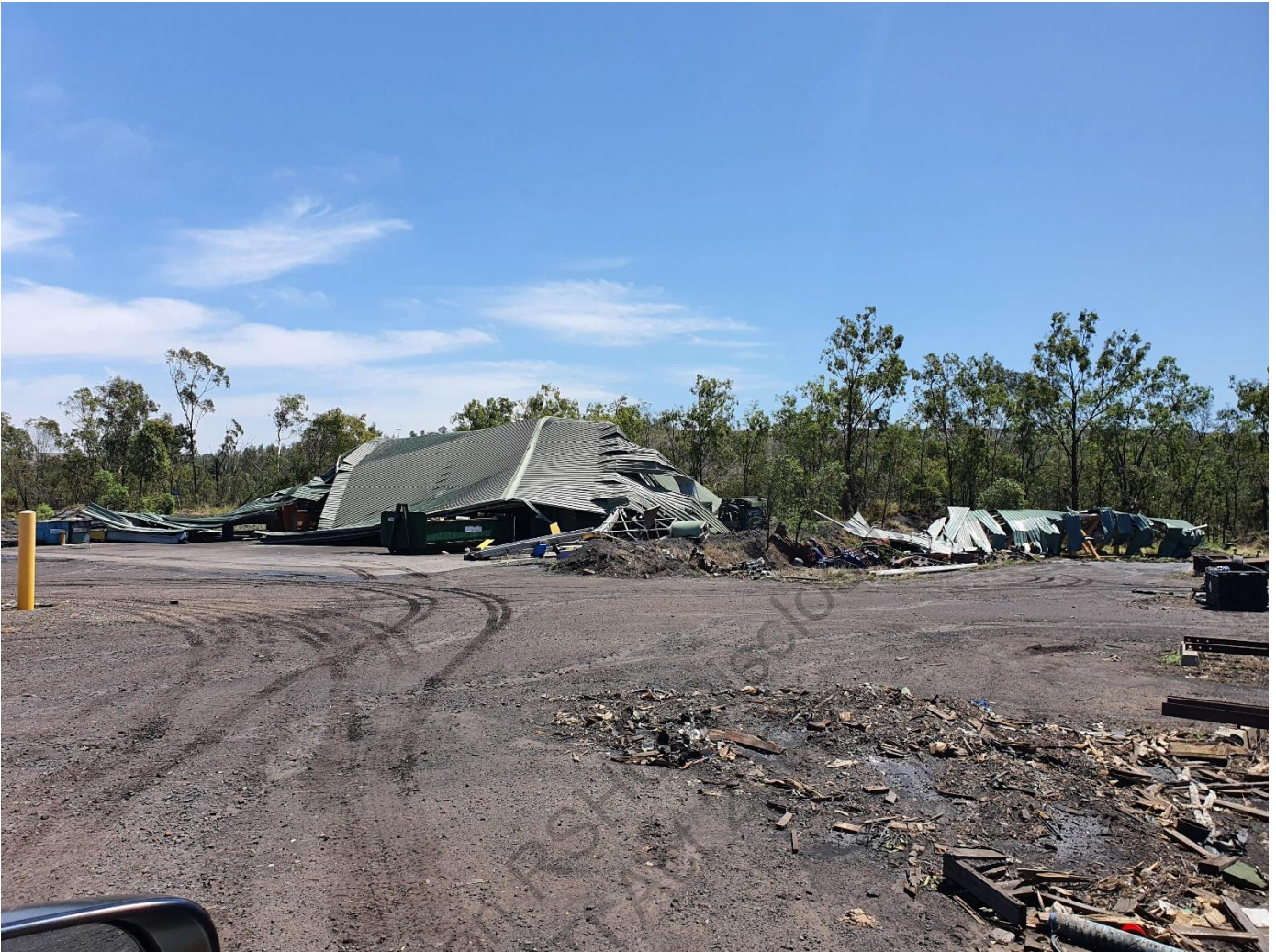
JJ Richards Shed
