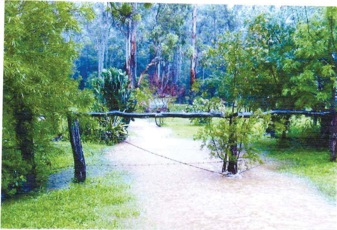
Photo 4 showing water flowing through property from culvert from roadway
