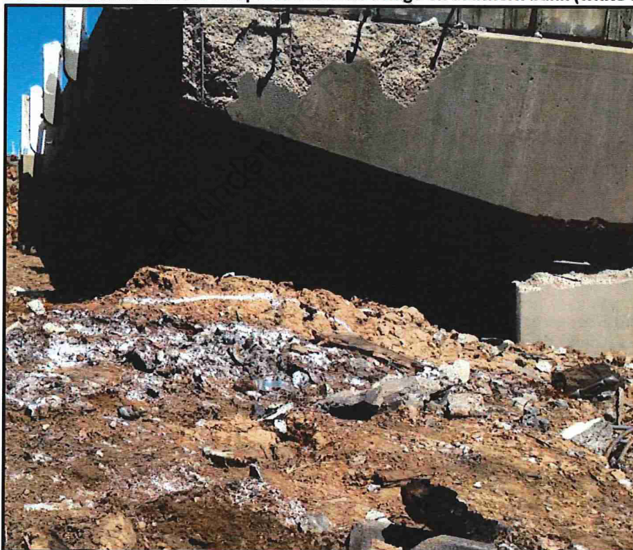
Figure 54 – Ammonium nitrate sample RB008 near bridge on southern bank (white areas).
